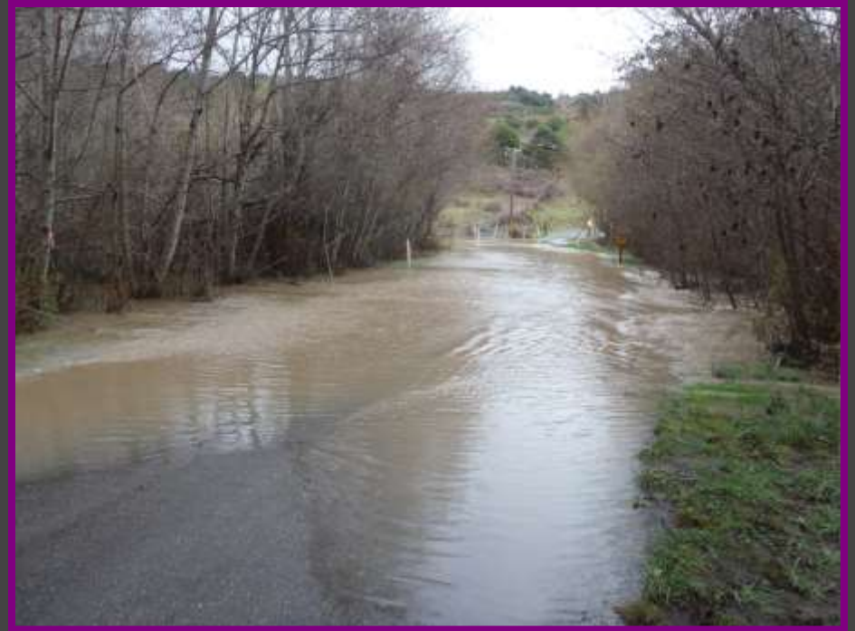
Willow Creek Crossing before replacement
