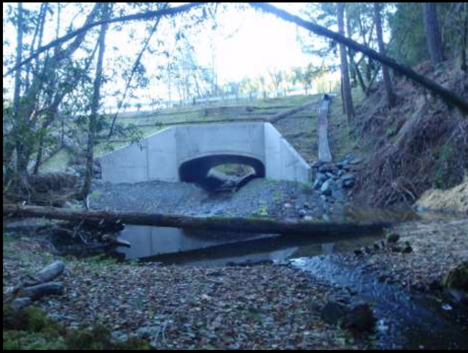
New bottomless arch culvert
