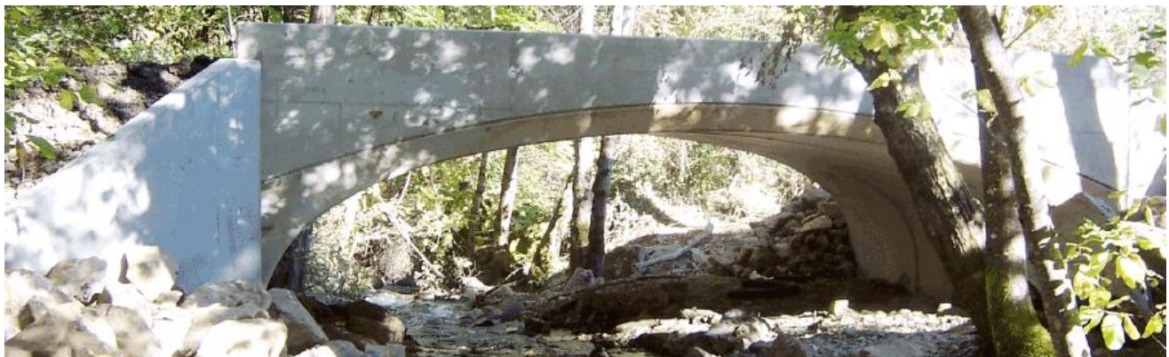
The Conner Creek Project will provide full passage for all life stages of coho salmon and steelhead by removing two culverts. Conner Creek flows directly into the Trinity River, a tributary of the Klamath River. Photo credit: Caltrout.org.
