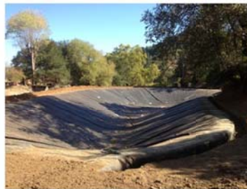
Installed Liner
