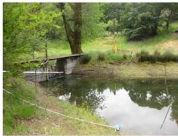
Existing On-Stream Flashboard Dam and Pond
