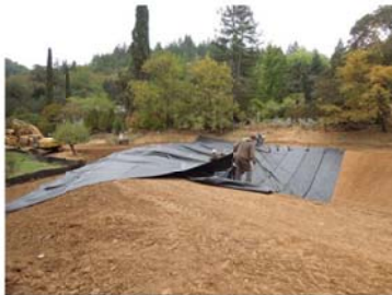
Liner Installation
