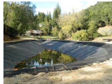
Completed Offstream Pond
