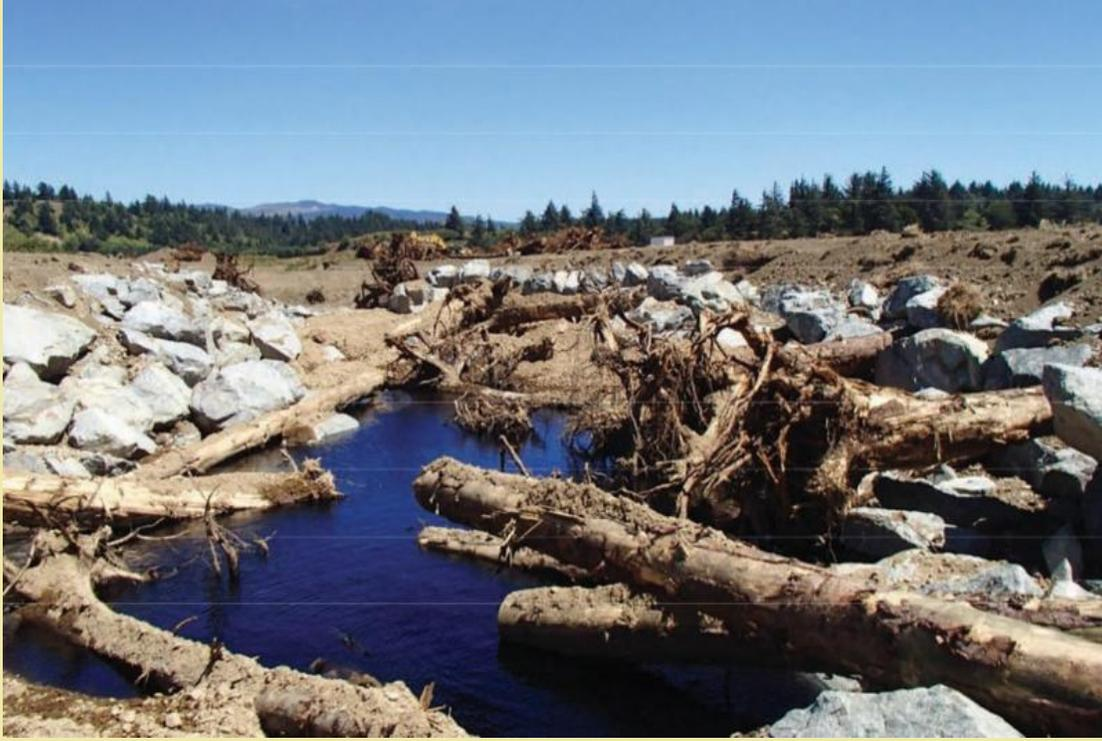
Fish passage-grade control rock structure. The rock features in the lower end of the alignment (pool-riffle) will be below groundwater, but they were designed and constructed to withstand southward migration of the Sixes River channel, which would change the overall slope of the lower Sullivan Gulch channel. Photo credit: Curry Watersheds Partnership.
