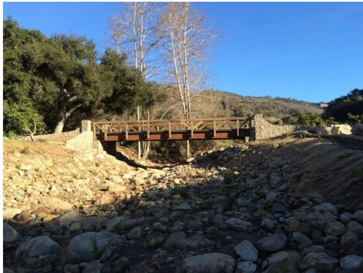
A project the California Fish Passage Forum funded in 2014, the Carpinteria Creek Fish Passage Project, was completed in 2015. The project addressed the last major barrier to steelhead in the watershed and opened up 1.27 miles of habitat by removing an undersized bridge and concrete channel to meet fish passage criteria for all steelhead life stages.
