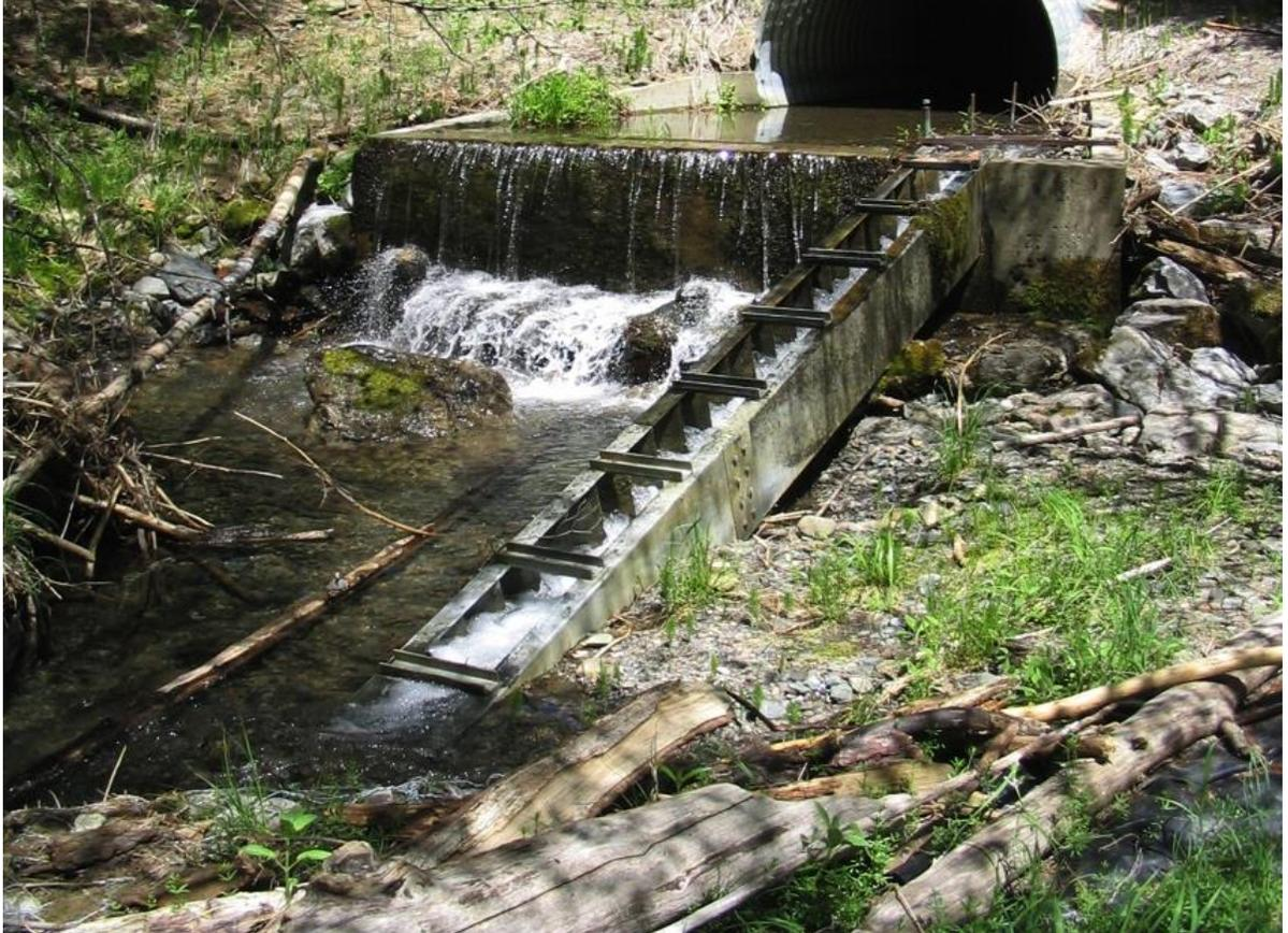
*Figures 2 and 3. The top photo features an example of a fish barrier that was remediated on the Shasta-Trinity National Forest. The bottom photo features the solution to the barrier—an open-bottom arch composed of natural streambed. This barrier remediation project created newly accessible habitat for Coho Salmon, Klamath Mountain Province steelhead, and Pacific lamprey. Photo credits: Shasta-Trinity National Forest.*
