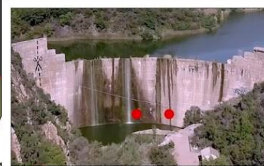
• approx location of low level outlets
