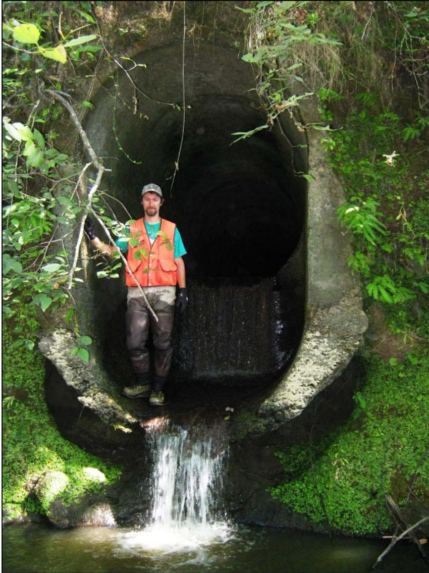
**Figure 8.** Two-stage drop at the outlet of site #NWPRR-243.38, photo taken on 8/17/11.
