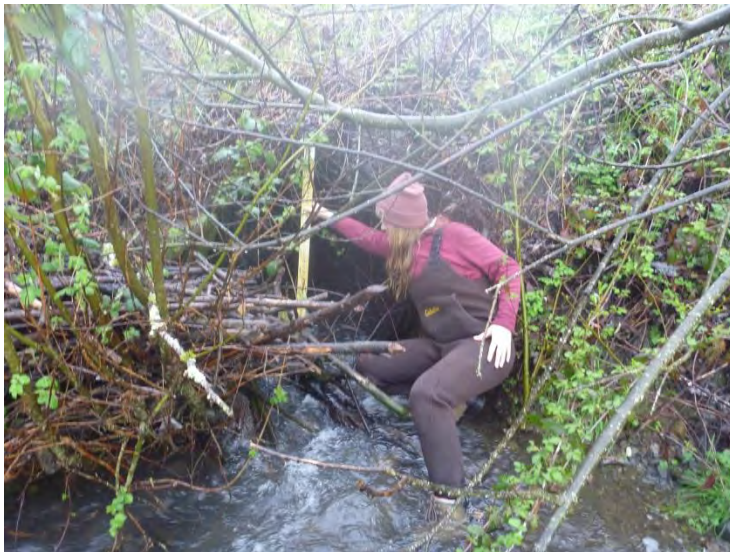
Figure 19. Outlet of one of the four culverts that comprise Crossing 4.
