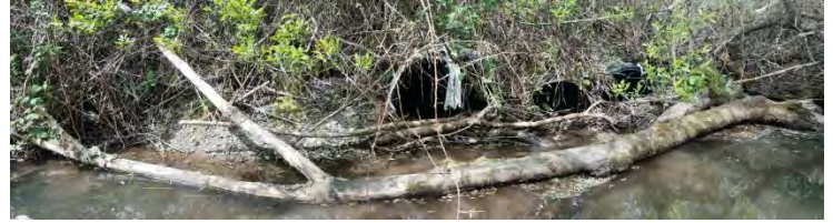
Figure 20. Inlet of 4 culverts that comprise crossing 4.
