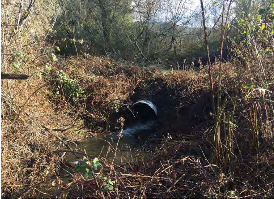
Figure 2-7. Crossing 1 outlet and shotgun scour pool. View looking upstream.
