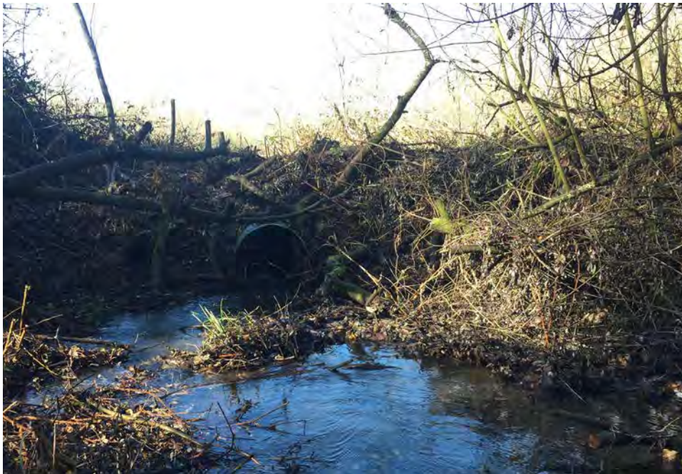
Figure 2-8. Crossing 1 inlet. View looking downstream.
