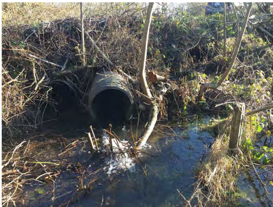
Figure 2-17. Crossing 4 outlet. Two primary pipes visible in center-left. Other two pipes obscured in blackberries to the right. View looking upstream.
