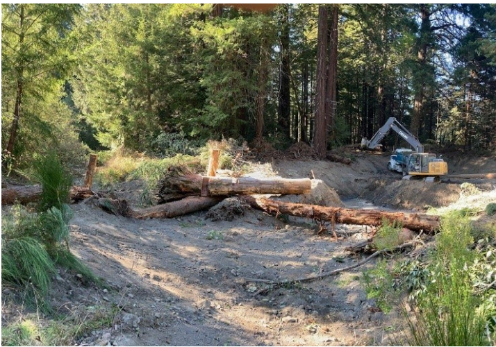
Photo 3a (top) shows the side channel pre-construction. Photo 3b (bottom) shows the completed Venturi structure, inlet jam, and entrance to the alcove situated in the existing side channel. Photo 3a was taken 9/27/22 and 3b was taken 10/11/22
