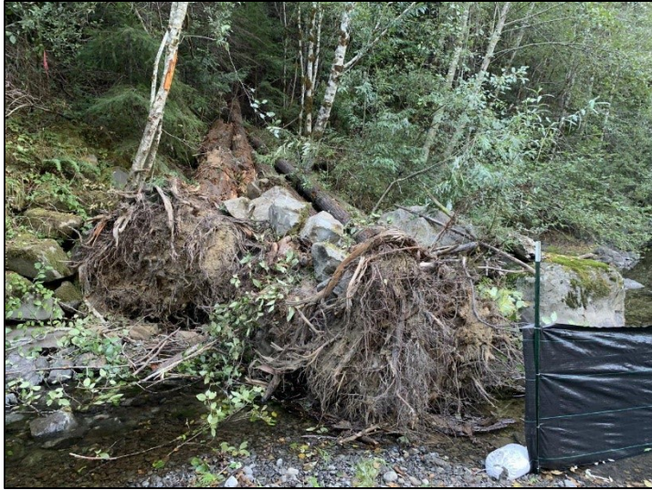
Photo 2 shows the constructed deflector jam (10/6/22).
