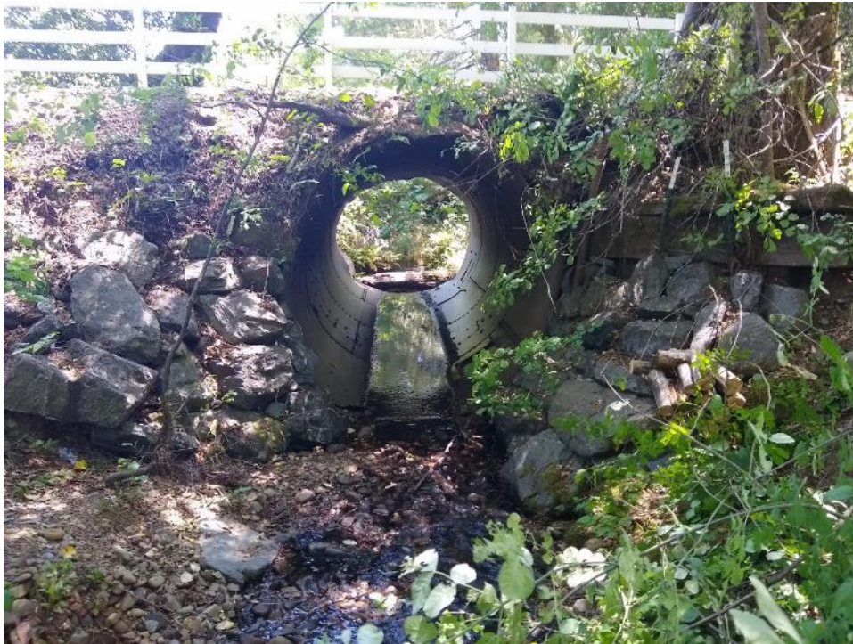
Figure 2-9. View looking downstream through Culvert 2. Note thin road base cover over culvert crest. Large diameter oak tree (right) is within the extent of disturbance for any alternative.
