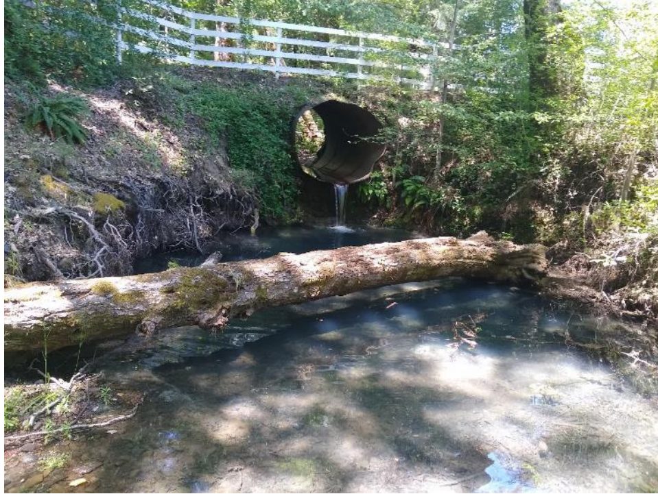
Figure 2-10. View looking upstream into the outlet of Culvert 2; impassable plunge visible (center). Evidence of scour and increased erosion rates are visible. Base of downed tree indicates historic location of bank.
