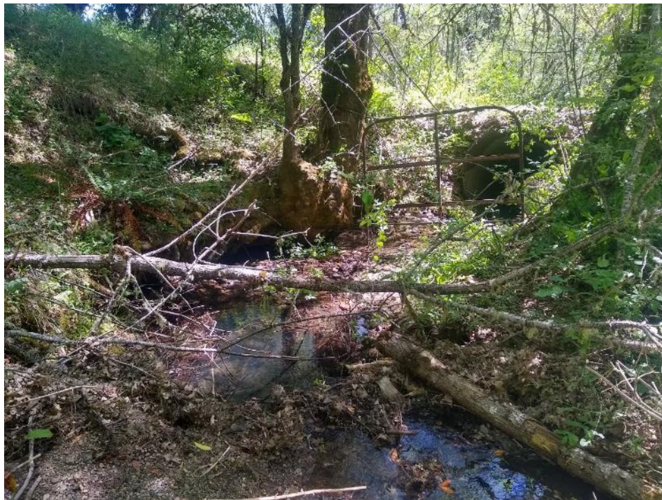
Figure 2-4. View looking downstream into the inlet of Culvert 1. Note strong bend in stream geometry immediately above inlet and large bay tree with under-cut roots.
