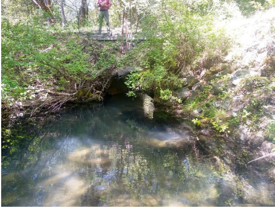
Figure 2-5. View looking over the scour pool, upstream into the outlet of Culvert 1. When the culvert crest elevation is compared to the previous figure, the steep slope is evident.
