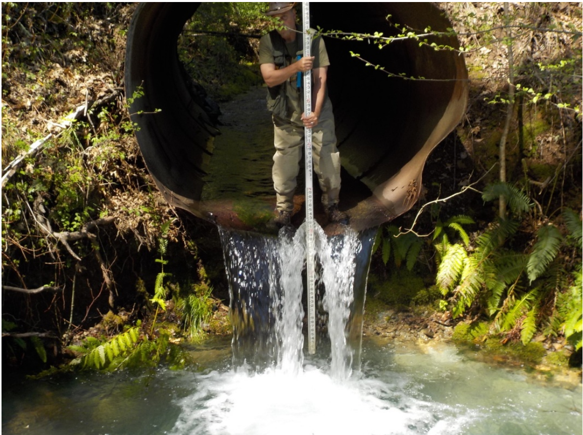
7 - Upper Culvert (#2), 3 foot drop to surface of pool, looking upstream from MC
