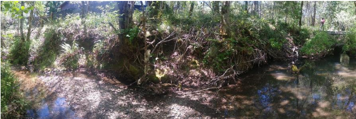
Figure 2-6. A roughly ~180-degree panoramic view of the downstream channel condition. Flow is from the outlet of Culvert 1, on the right, through the scour pool, and across the gravel bar to the left. Residence visible in background.
