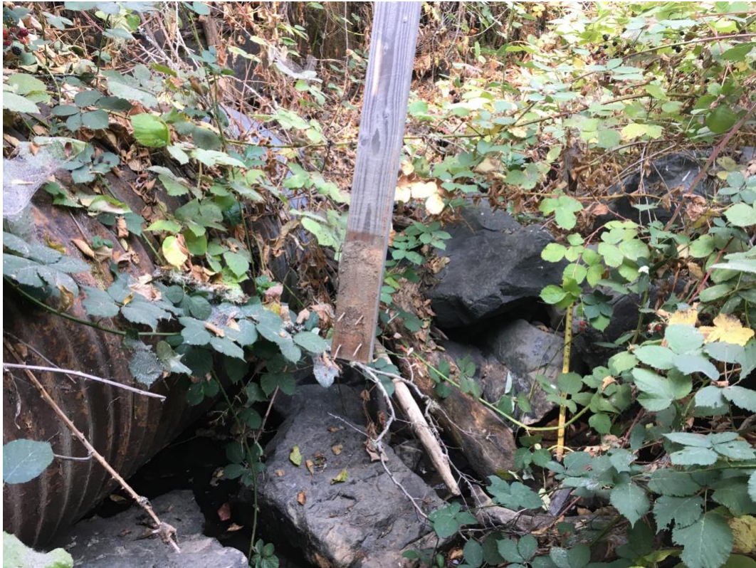
Looking upstream at culvert inlet and rock weir.
