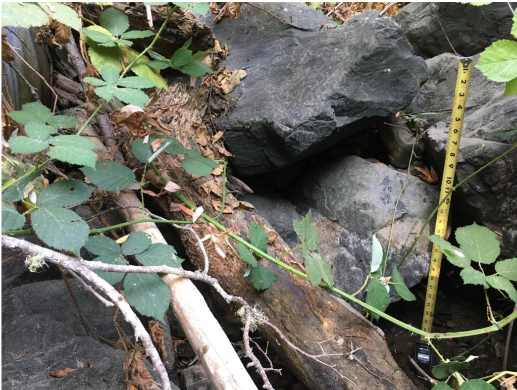
Looking upstream at rock weir with measuring tape showing plunge.
