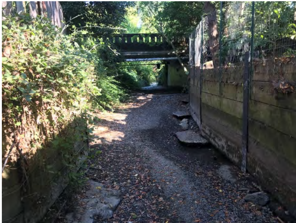
Looking downstream towards the bridge crossing, adjacent wall footings are noticeably eroded. (Sep. 2019)
