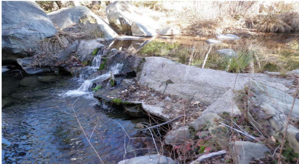
Figure III-1. Lion Creek check dam before removal, looking upstream from left bank at small (3.1 feet high). Lion Creek check dam was removed in October of 2014. Photo courtesy of CCC Camarillo.
