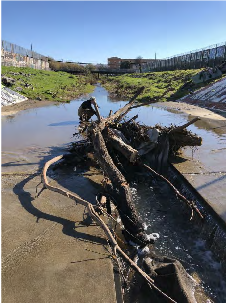
Photo 3 - Woody Debris Blocking Fish Ladder Following January 15-17 Runoff Event - January 24, 2019.
