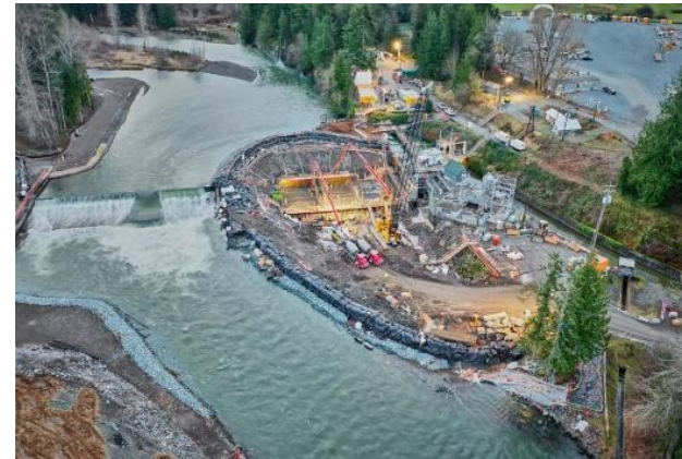
Mud Mountain Dam Fish Passage, WA
