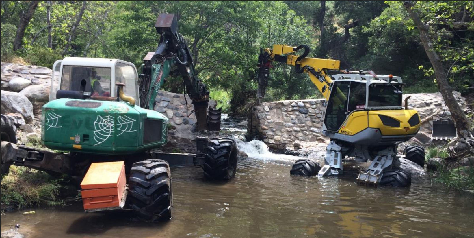
Spider excavators remove a dam on San Juan Creek in Cleveland National Forest. Photo: Julie Donnell, USFS
