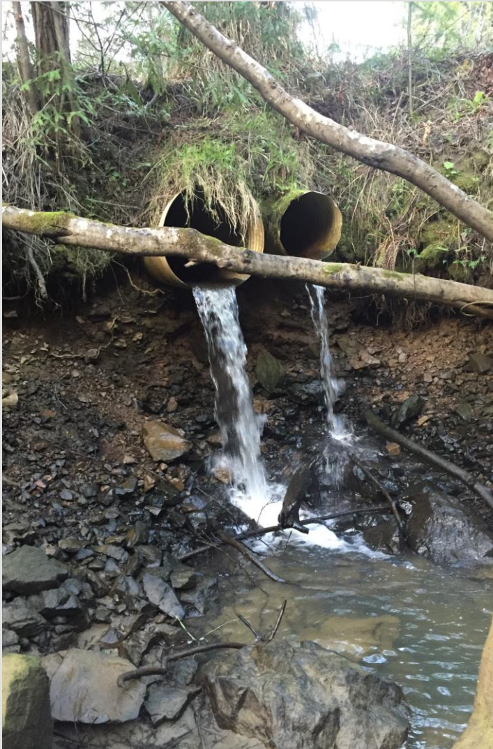
Dry Dock Before (L)
