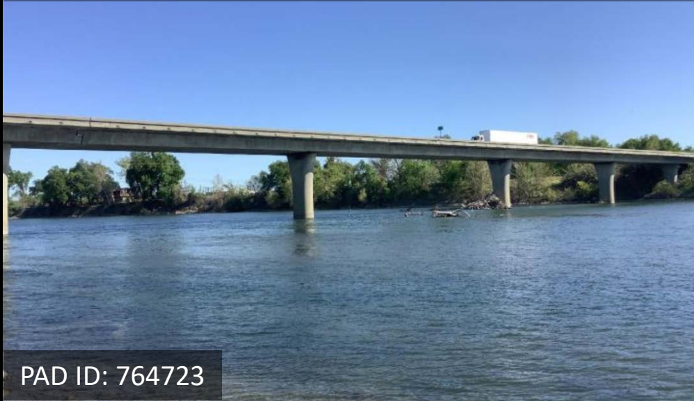
Hwy 32 over the Sacramento River
