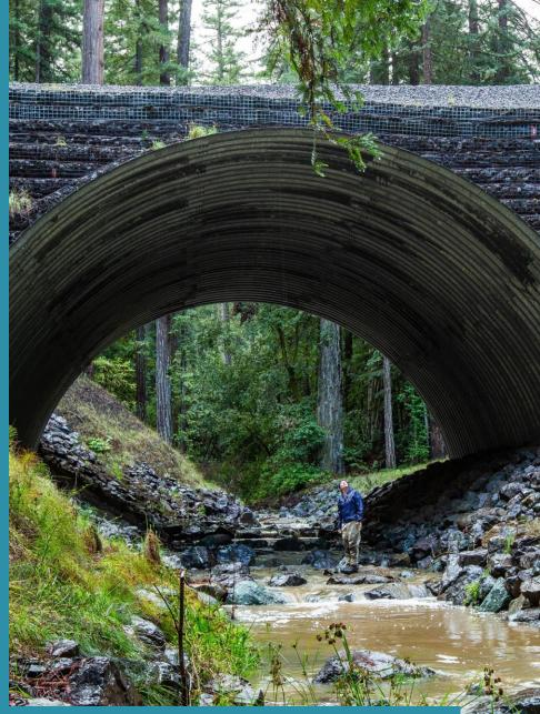
A 2019 Project lead by Trout Unlimited to install a large bottomless culvert at the Skunk Train crossing of Noyo River, east of Fort Bragg.
