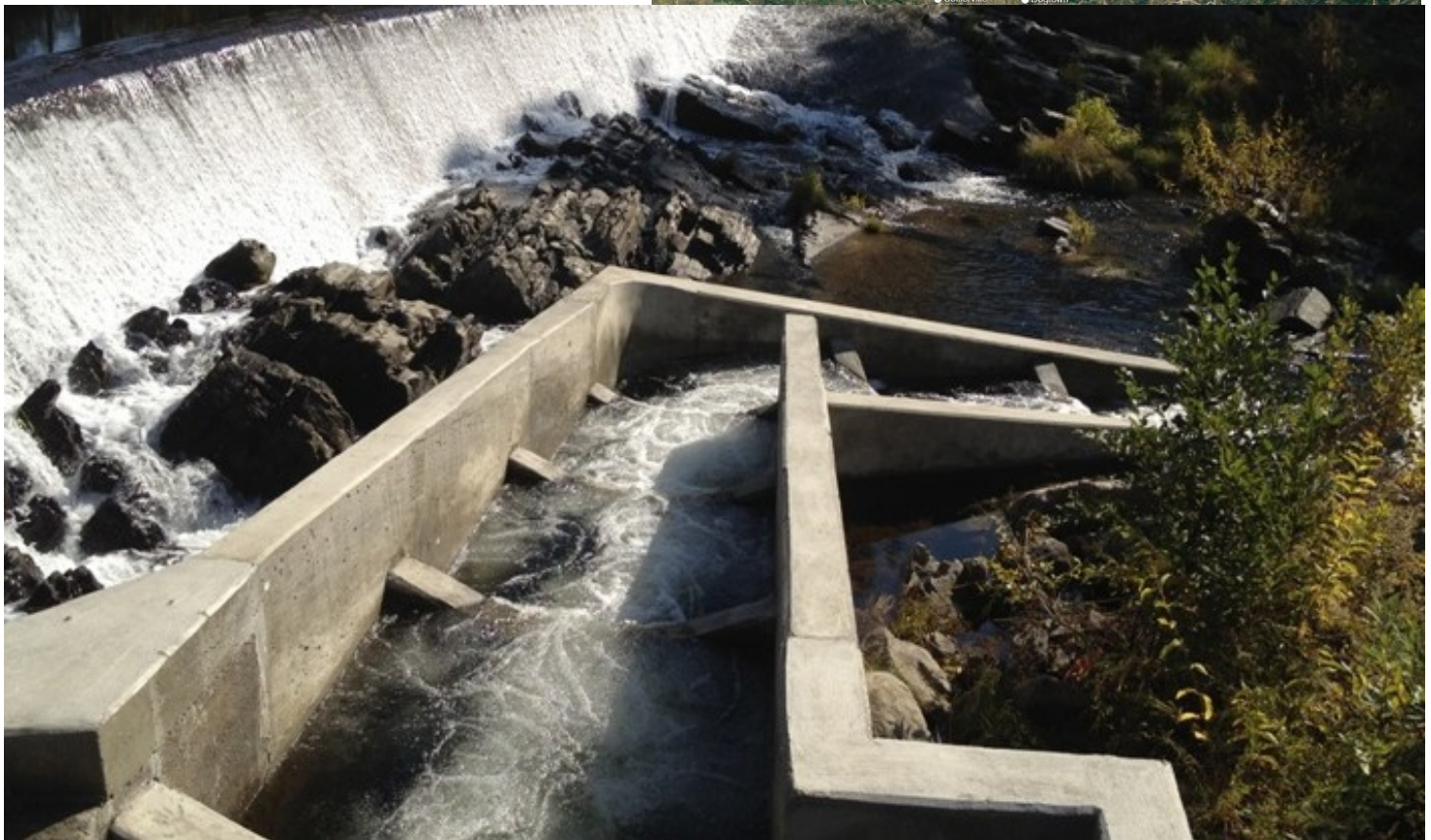
Figure 1. Map showing location of Granlees dam project (right). Figure 2. The completed project provides a runway for fish to migrate upstream.
