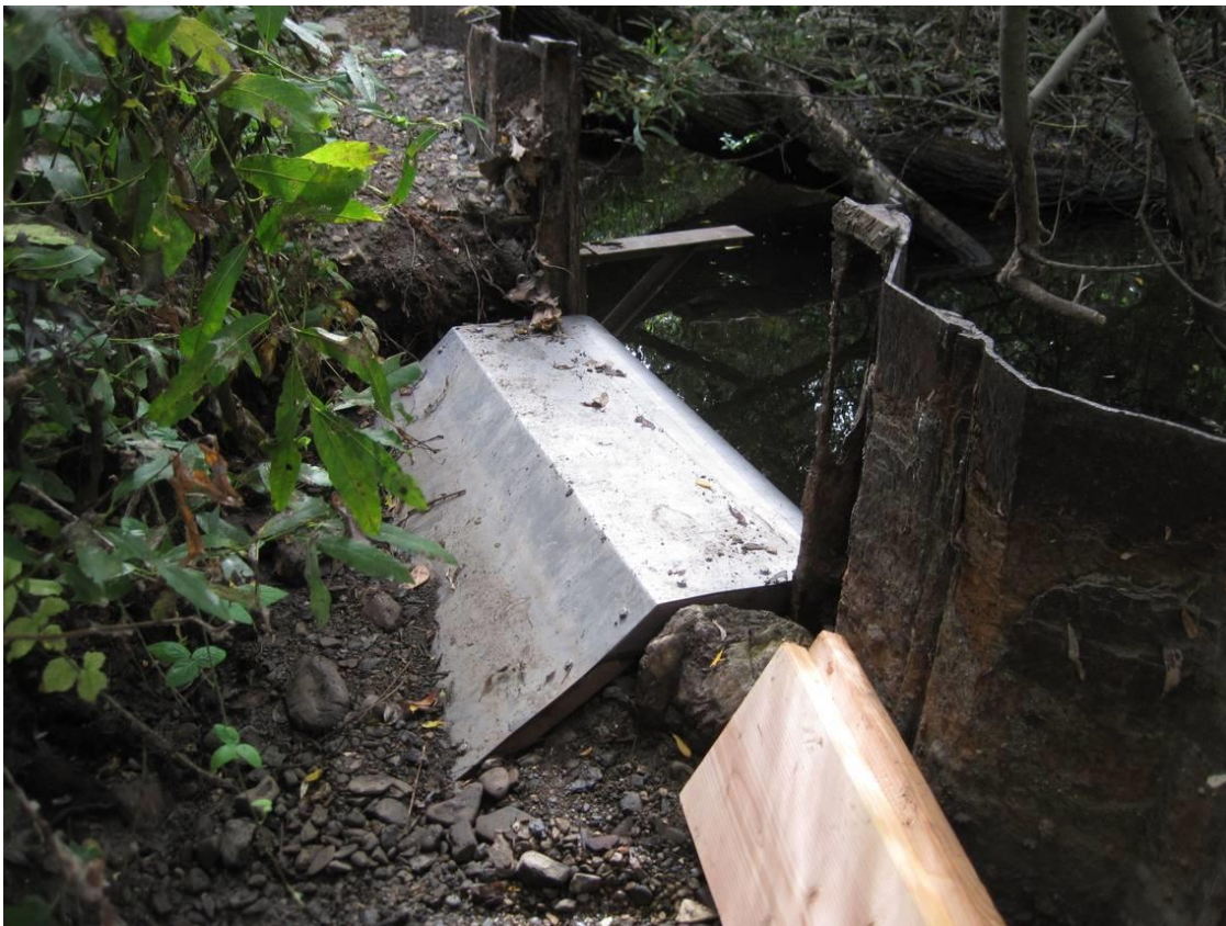
Lamp Ramp installed near the mouth of San Luis Obispo Creek in 2013. Photo courtesy of City of San Luis Obispo.
