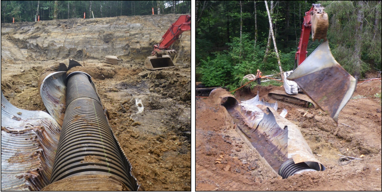
Figure 2. Deep road fill was excavated and stockpiled, the failing culvert was carefully removed allowing for reuse of the temporary plastic liner. Degree of failure of the culvert is visible at right
