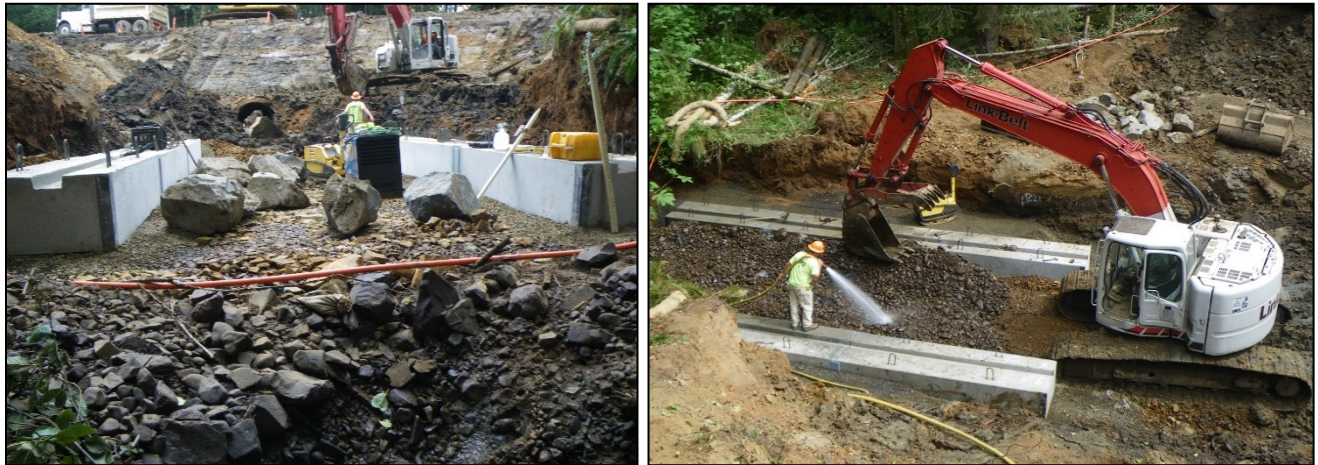
Figure 4. Proper sizing and installation of streambed materials is critical to success, including washing in fine sediment to ‘seal’ the streambed features. This ensures that when flow is returned to the channel, a low flow channel is maintained rather than flow going subsurface.
