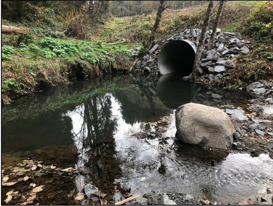
Figure 2. Pass creek post retrofit, showing boulder weir and roughened channel installed downstream of culvert to back-water outlet, eliminating perched condition and allowing fish and lamprey to swim into the culvert without jumping.
