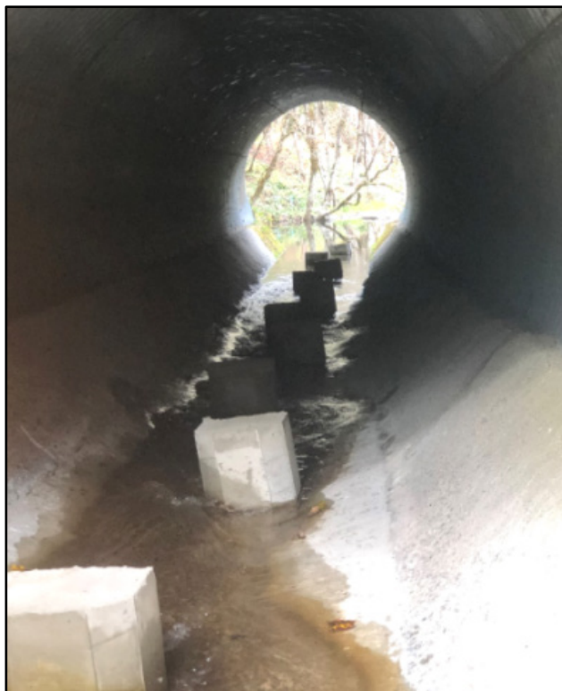
Figure 3. Post project photos. Fish blocks installed throughout the invert of the culvert to provide localized velocity reduction and resting areas for migrating fishes.
