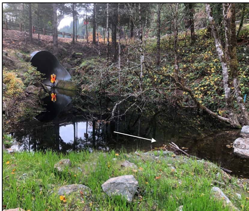
Figure 4. Post project photo: new boulder weir and roughened channel (designated by arrow) installed downstream of the culvert.
