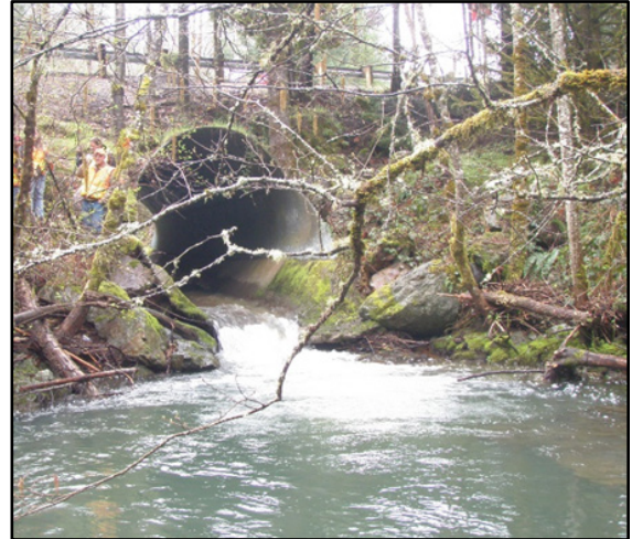
Figure 1. Pre-retrofit photo: culvert is perched above the water surface and undersized.
