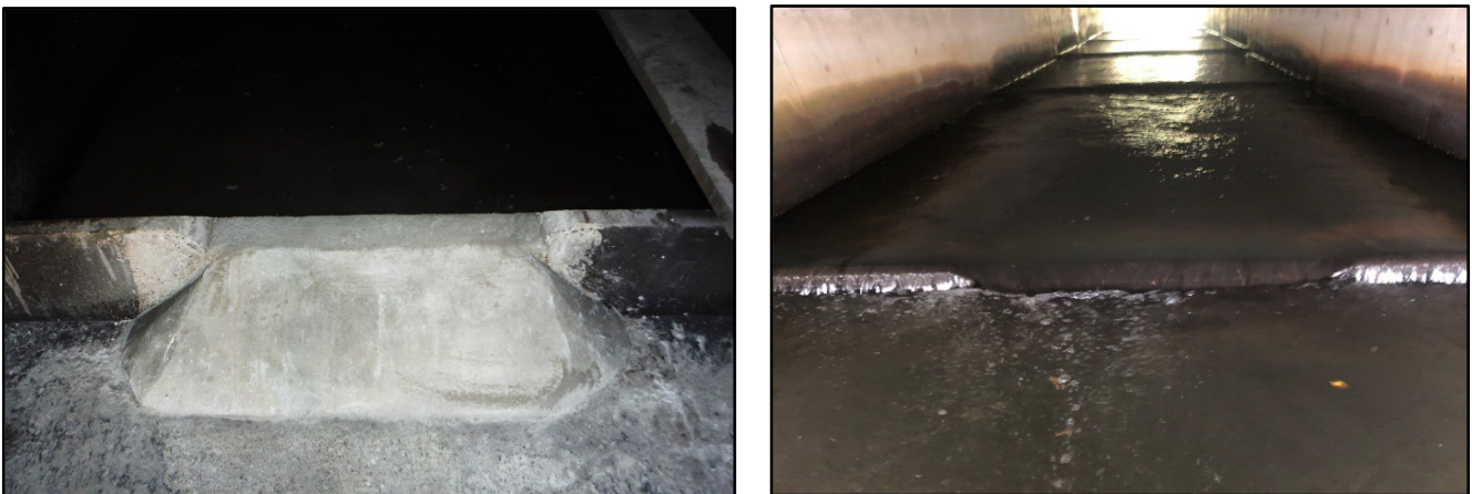
Figure 3. Photos of the modified baffle and ramp in dry and watered conditions. Middle portion of the baffle was cut down and a ramp was installed on each side of that cut to provide lamprey with a continuous attachment surface.
