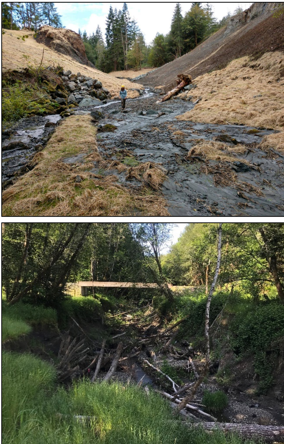
Figure 3. Pilot channel shortly after completion (top). Project site after first winter, showing natural recruitment of large wood. Constructed log jams will be placed in 2020 using the recruited wood in addition to larger pieces.
