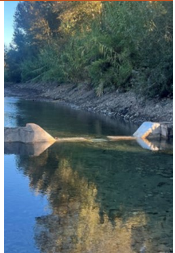
Notch at Foster park during low flow conditions
